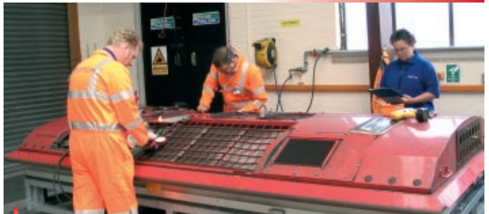
HVAC (Heating, Ventilation & Air Conditioning) module testing after repairs
