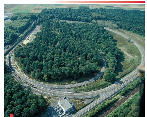
The test center at Valenciennes, France
