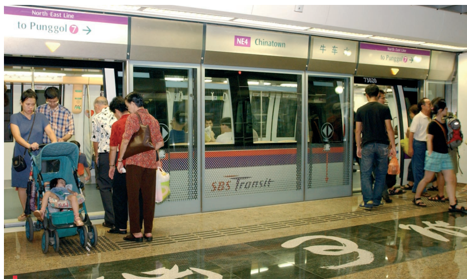
Precision stopping: when the train stops at stations, the alignment with the platform screen doors is highly accurate
