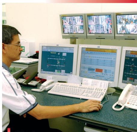
Automatic train supervision from stations thanks to our ICONIS DMS system
